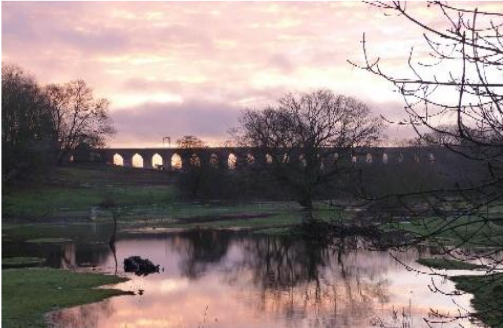
Digswell Viaduct & Digswell Lake
